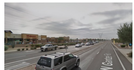
Regional Connection Gantzel Road, Pinal County
